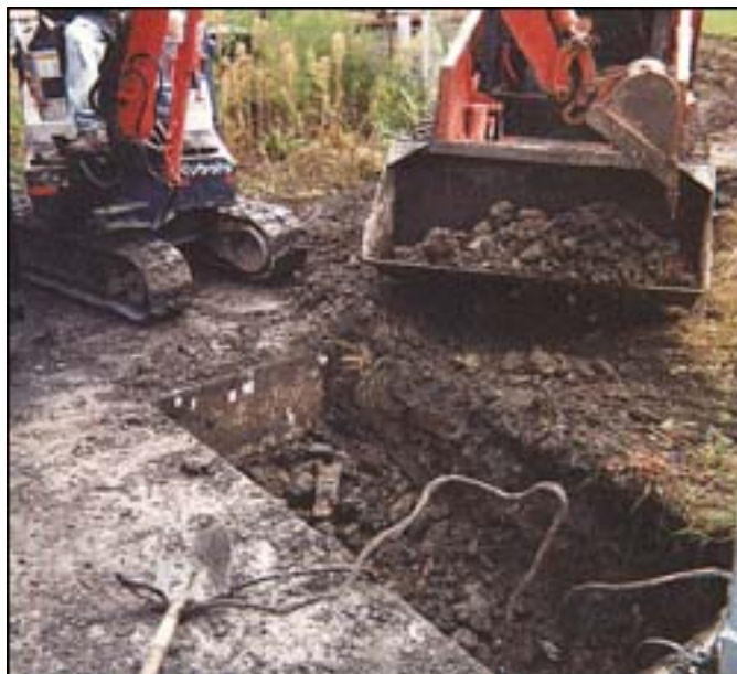
PCB site clean up.
